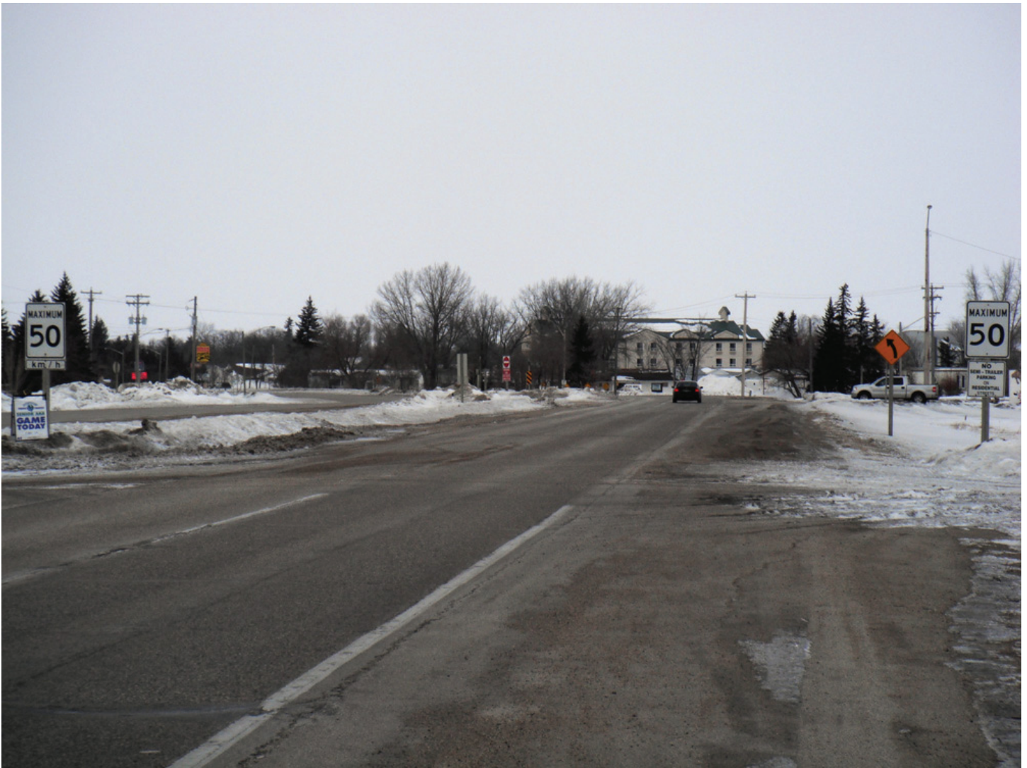
Photo showing MUTCD compliant speed signs on a Province of Manitoba roadway – signage is on both sides of the road, at proper height for driver visibility and is much larger than City of Winnipeg signs.
