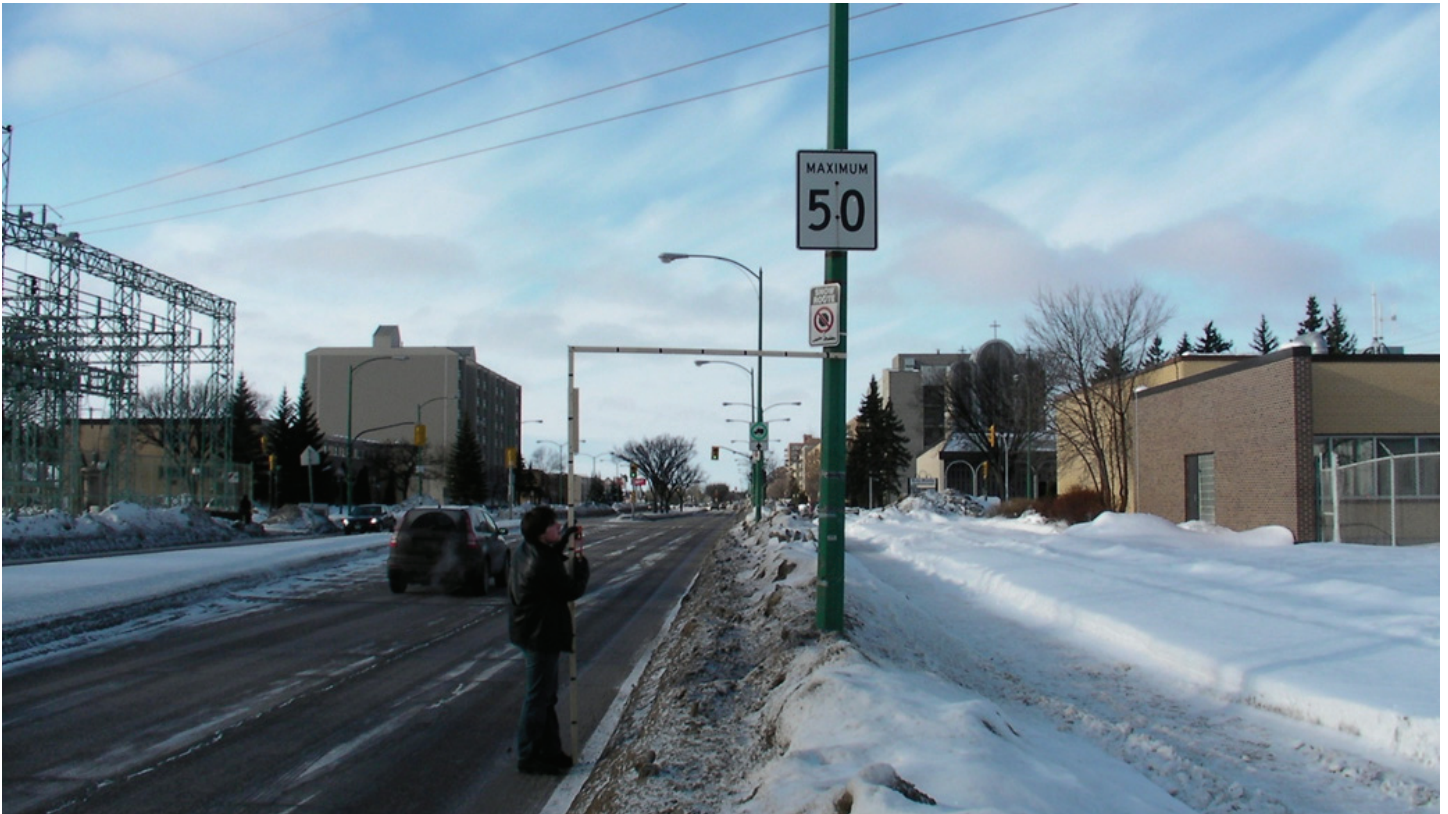
Photo of MUTCD height standard applied to the single reduced-speed limit sign on westbound Grant Ave. approaching camera intersection at Wilton St. The sign significantly exceeds the 3.0 meter maximum height.
